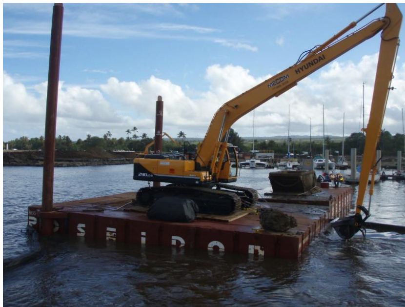
Figure 2. Photo of dredge operation during 2009 maintenance dredging.
